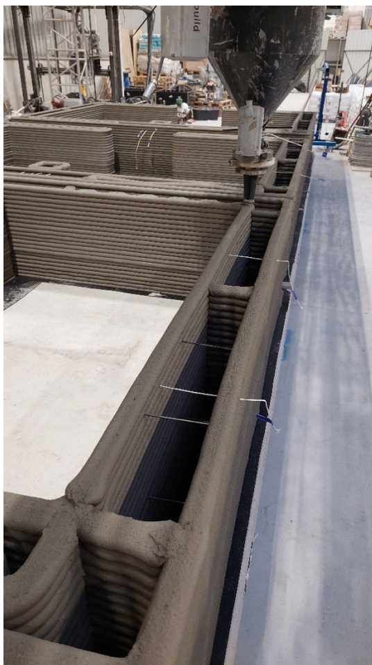
Fig. 4. Printing of houses (reinforcement and thermocouples are visible)
