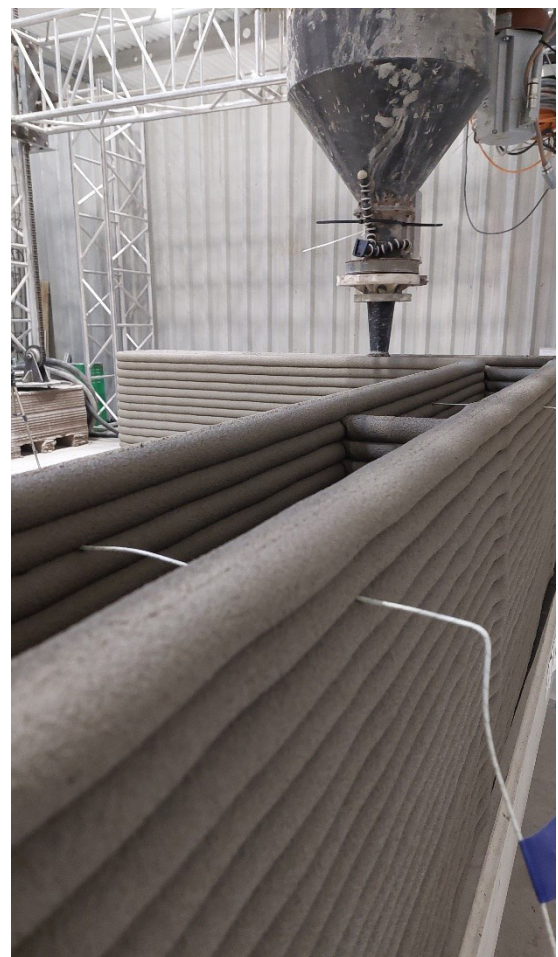
Fig. 4. Printing of houses (reinforcement and thermocouples are visible)
