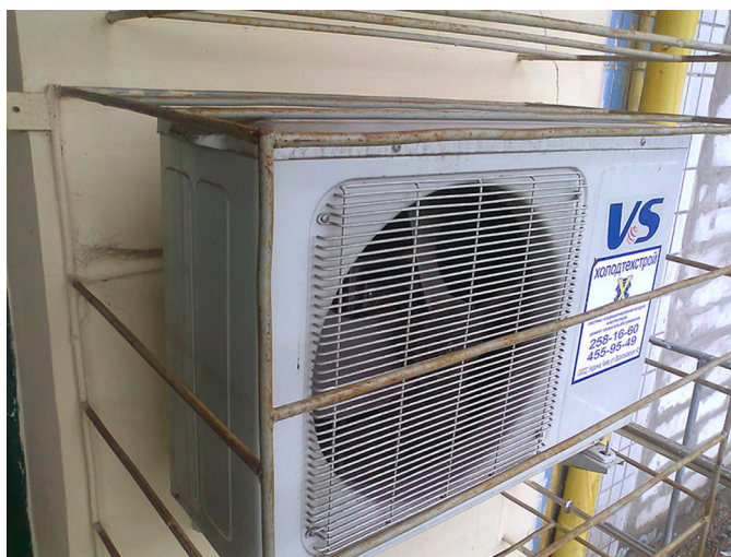
Fig. 5. External unit of air-conditioning system of Split type [6]
