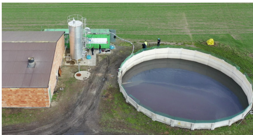
Fot. 1. Pilot biogas plant: a) site of biogas plant (a view [Photo by G. Wałowski] – from right: fragment of pig house, mono substrate flow reactor for methane fermentation of pig slurry together with the installation for production of agricultural biogas, lagoon for post-fermentation product; b) adhesion bed, made from vertical pipes with coarseness of 80 μm, transported to the inside of fermentor – a view [Photo by G. Wałowski].
