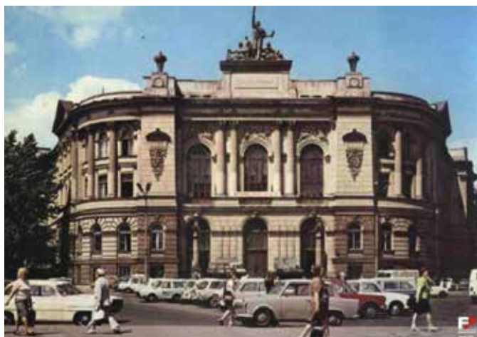
Fig.7. The main building of Warsaw University of Technology in 1975, the site of the Faculty of Geodesy and Cartography (Source: warszawa.fotopolska.eu/310159.foto.html)
